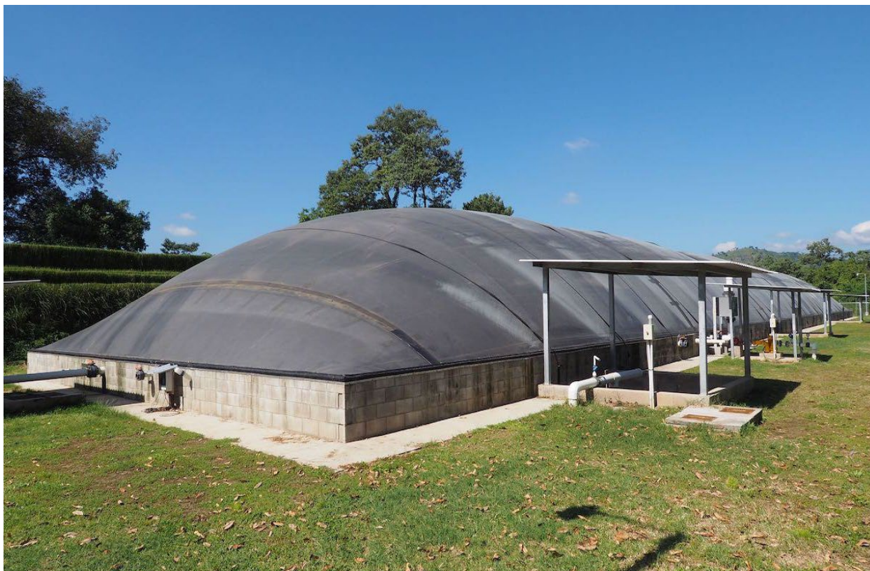
Figure 7: Poultry Lagoon Anaerobic Digester
